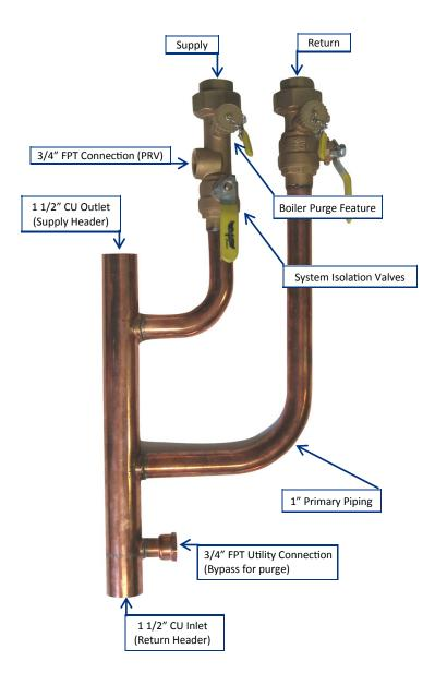
Re-designed manifold with 1" copper primary piping spaced at 6" on center
