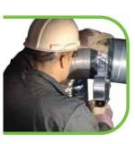
The TapeMaster is the industry's first and only aluminum foil tape dispenser, engineered for removal of the paper release liner from foil tapes with ease. It conveniently rolls the waste paper onto a take up reel for easy disposal, eliminating thousands of little pieces of scrap from the job site. The built in squeegee helps to apply and smooth the foil tape in one motion, leaving a professional look to your job. The TapeMaster saves
